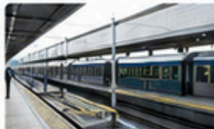
Transportation Hubs Passenger information and emergency messaging
